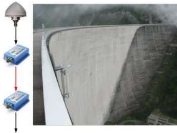
GPS antenna cable extended by a ViaLite GPS over fiber link
